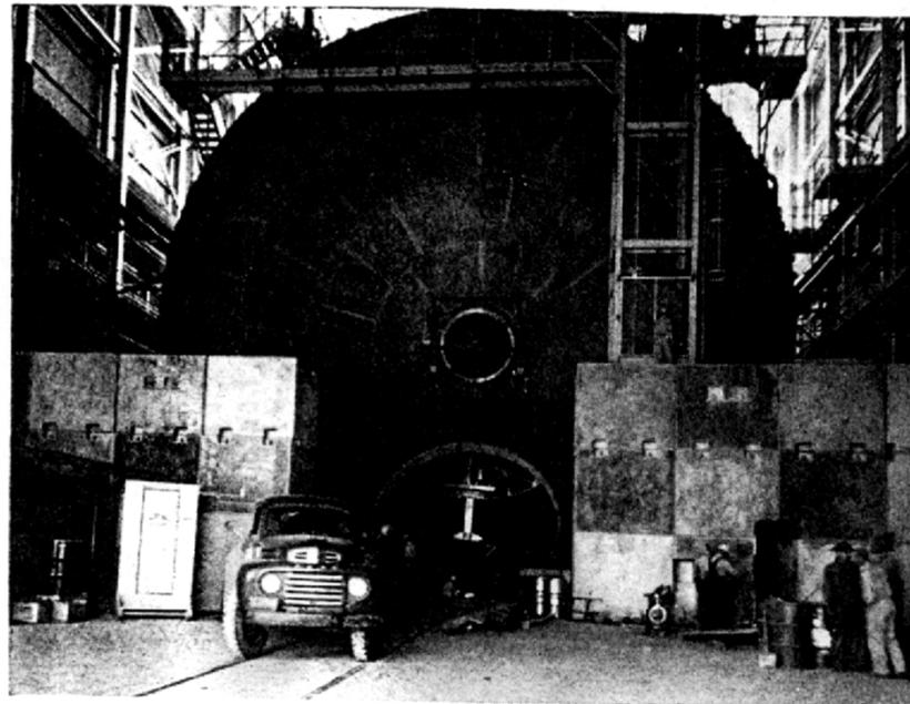
**BIGGEST VACUUM VESSEL** ever built, 60 feet in diameter and 87 feet long, housed Materials Testing Accelerator. Men and truck in photo show comparative size. Door 20 feet in diameter, opened at tank's bottom, admitted rail car handling drift tubes. Concrete blocks like those seen formed unbroken wall of shielding while the accelerator was running.
