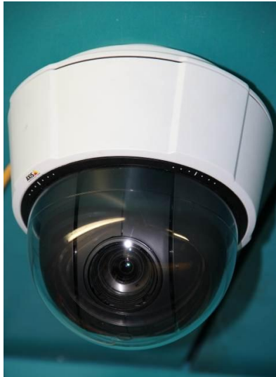
IP camera in bunker
